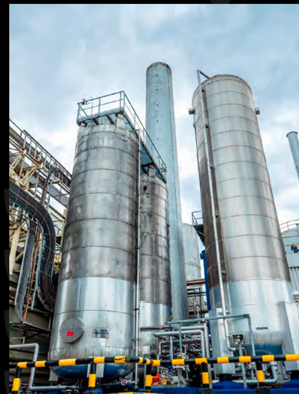
Photo: CO 2 Storage Tank in TBL Plant Dar es Salaam
